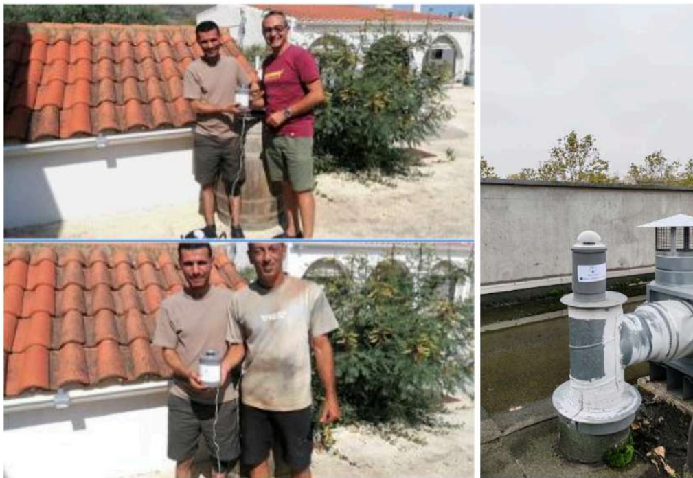
Figure 30: Installation of low-cost skycamera
